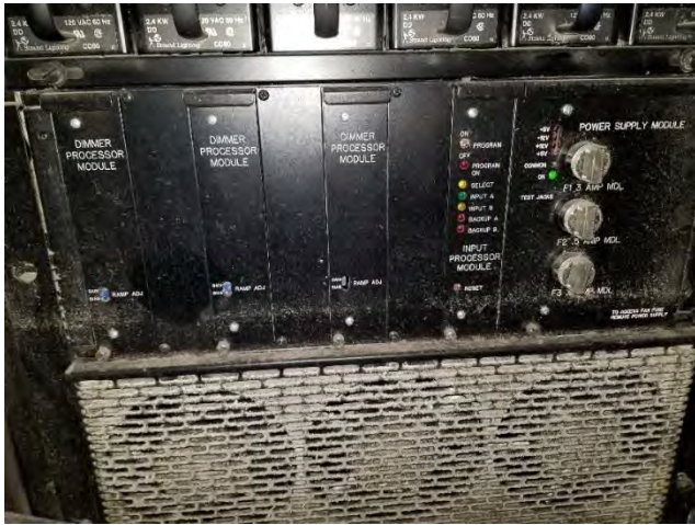
Front, bottom of Strand rack with the original analog controls. Rack can be upgraded with digital controls in one day allowing relay and constant power modules to be added for LED fixture power.
