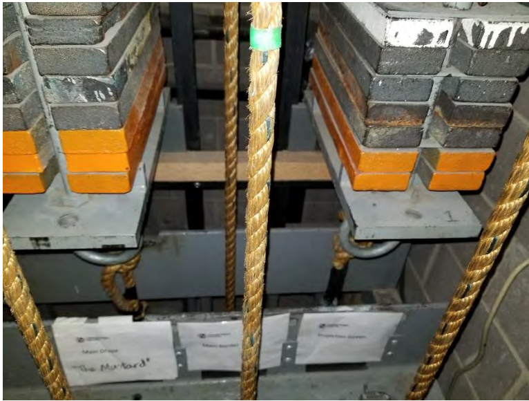
Bottom of arbor, running rail and operating lines
