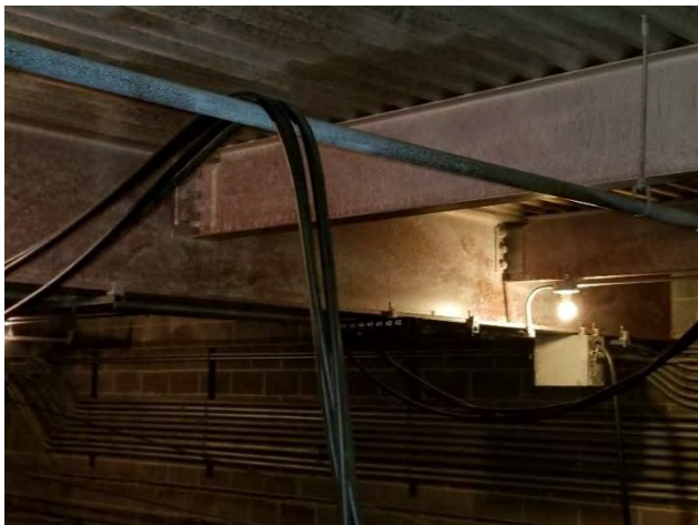
Circuit cable lying over sprinkler pipe at the grid
