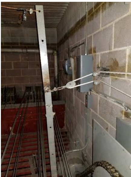
Fire curtain arm under tension is released to fall when release line is pulled at the stage. The end of the arm is tied to circular weights that fall creating the momentum to start the curtain moving downward
