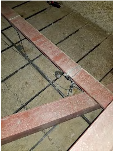
Speaker rigging is wire rope looped over the angle iron and secured together with wire rope clips. Hardware should be removed. Wire rope is not designed to bend in that manner
