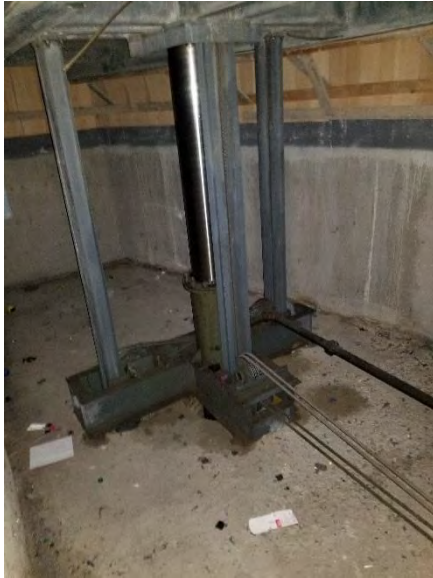
Underside of orchestra pit lift. Stage left side is fairly clean while the hydraulic fluid on stage right appears to be leaking. Rest of hardware appears in good shape
