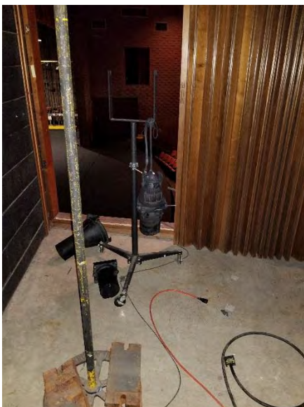
Picture of box boom area which is missing a chain or railing of some sort to stop a technician from falling into the audience chamber
