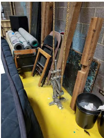
Rigging for rear storage area paint wall. Floor block on right is the control and the arbor shown on the left is the counterweight for the wall and canvas.
