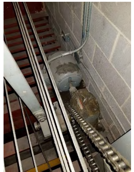
The fire curtain motor at the grid used to raise the curtain back into place. Motor can be used to drop the curtain in for service.
