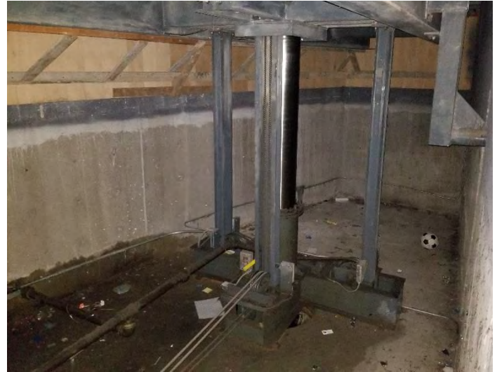
Underside of orchestra pit lift. Stage left side is fairly clean while the hydraulic fluid on stage right appears to be leaking. Rest of hardware appears in good shape
