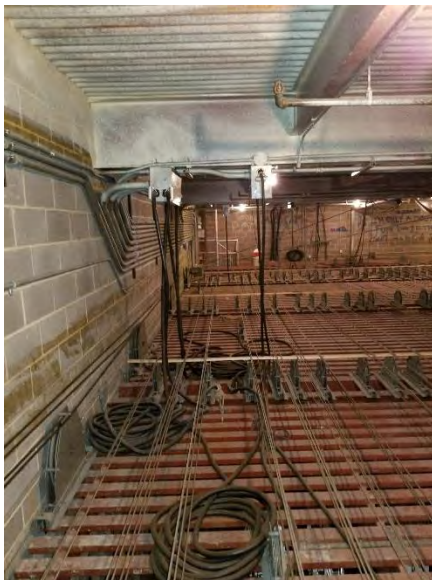
Original theatrical circuits in underhung junction boxes at roof beam. The box on the right needs new mounting hardware to secure it. Ungrounded SO cable lying on the steel grid.
