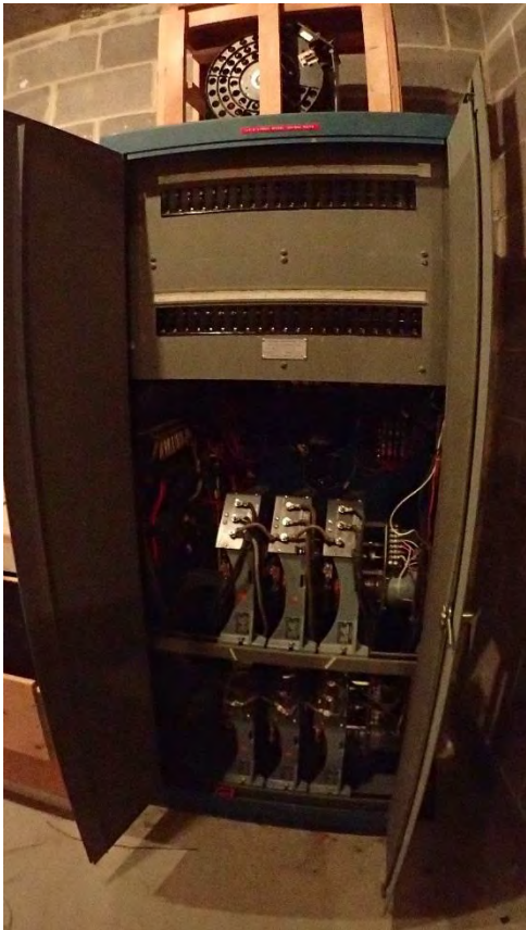
House light dimmer rack. 20A breakers feed into the 70A dimmers. Cabinet is located near the backside of the house right box boom.
