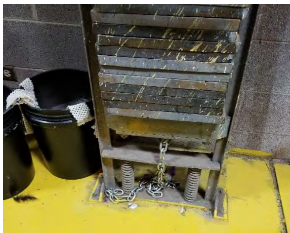
Rigging for rear storage area paint wall. Floor block on right is the control and the arbor shown on the left is the counterweight for the wall and canvas.
