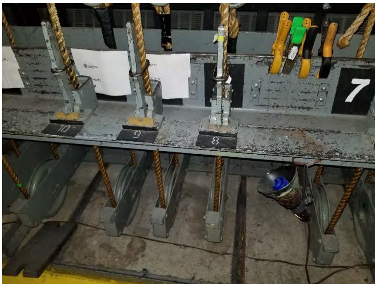
Original rope locks that are only designed to last 15-20 years
